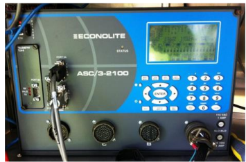
Traffic Signal Controller
